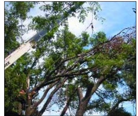
Fig. K: A climber has used the tie-in point on the crane to set two chokers on this partially broken, hanging tree top, descended to the break, and is positioning himself to prepare to make the cut (the climbing line will be removed from the crane before the cut is made; photo courtesy of Kramer Tree Specialists).
