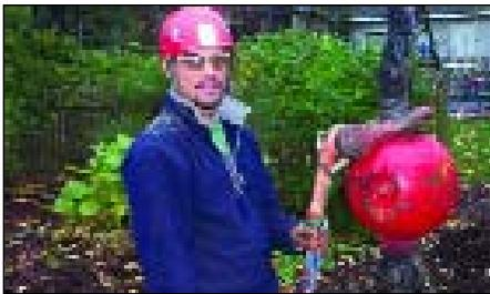
Fig. I: Another tie-in option is to place a large (here a 17 ton) shackle above the ball and thread a false crotch through the shackle. A carabiner is placed in the eye of the pin of the shackle and around both legs of the false crotch (photo courtesy of Norm Hall, The Care of Trees).
