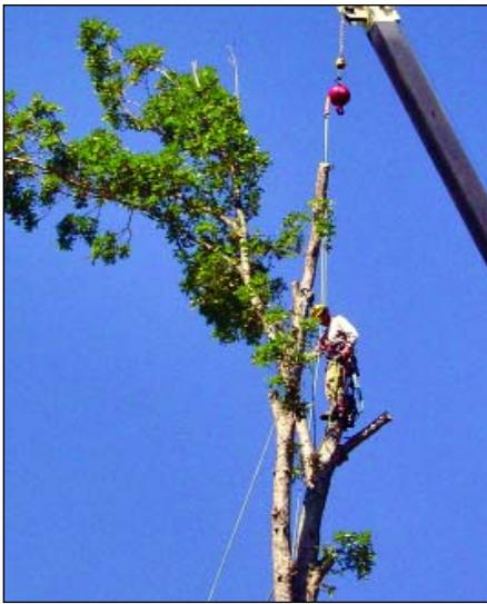
**Fig. O -** A climber using the crane as a tie-in point while he is rigging the tree using ropes, a block, and a friction device. If the tree had failed, the climber was safely suspended from the cable of the crane. Note that the anti-two-block system is unaffected by the tie-in system.
