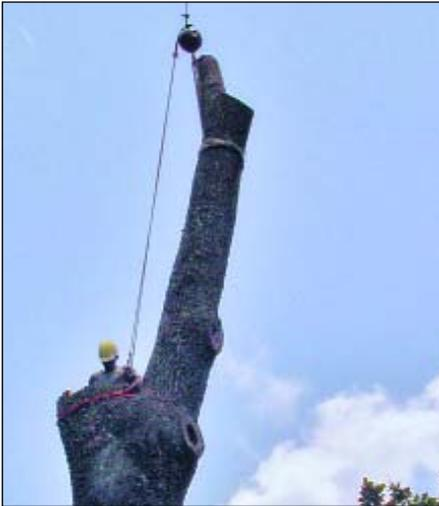
**Fig. M:** *This climber has set a choker on the top of the spar and descended to the point where he will make his next cut. He is positioning himself at a large branch union, something that would be much more difficult if he were descending on just his spikes and a lanyard.*
