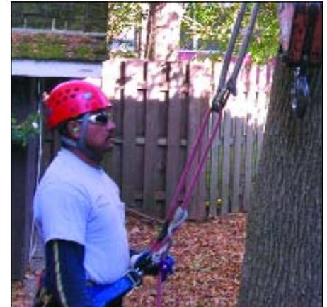
**Fig. G:** *Another way to thread the climbing line is to place a rated carabiner (one which is self-closing and self-locking, with a minimum tensile strength of 5,000 pounds) in the false crotch right next to the small ring (photo courtesy of Todd Kramer, Kramer Tree Specialists).*
